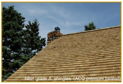
ACQ pressure treatment is available to enhance the natural durability and resistance of cedar in particularly demanding situations. Copper and quaternary compounds are effective fungicides and termiticides. Together they provide enhanced protection against a broad spectrum of decay fungi, borer and termites.
